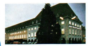
Plant at Steyr/Austria
