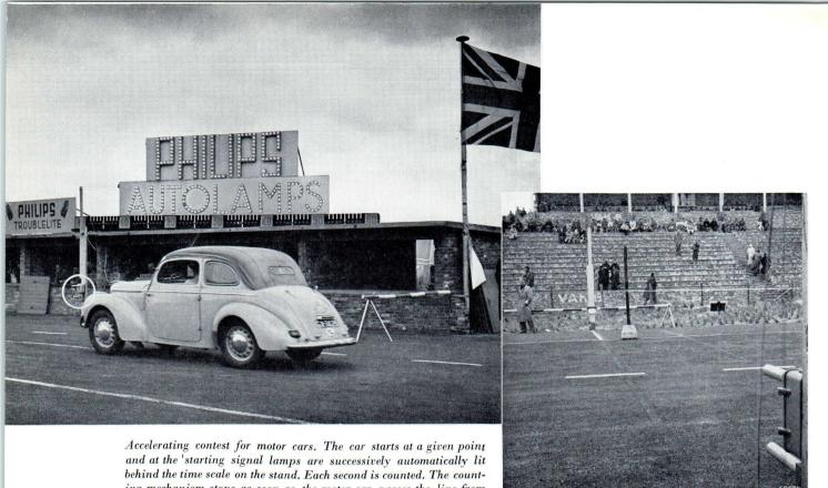
ing mechanism stops as soon as the motor car passes the line from the light projector to the phototube and the public can easily read the time made by each car.
