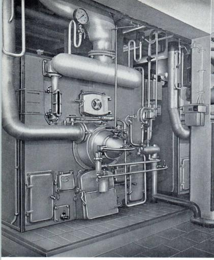
Flame control with phototube. A phototube "watches" the fire in the boiler. When the fire extinguishes the fuel supply is stopped and an alarm signal is given, so explosion is prevented.
