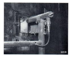
A simpler method of mounting a phototube system for flame control.
