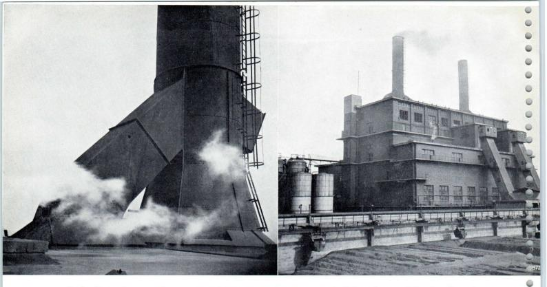
Smoke detector in use with power plant (right). On the left photograph the light projector and the phototube receiver are to be seen on both sides of the funnel-uptake.
