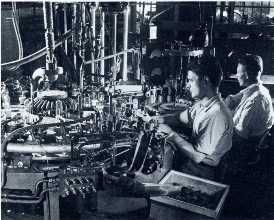
Fig. 54. Rotating pump and sealing machine for radio tubes.
