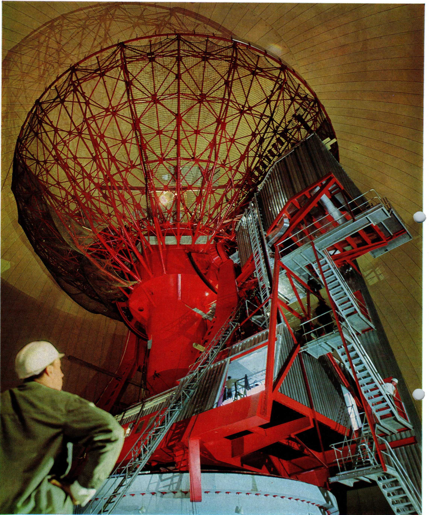
Antenna system of Raisting earth station. Dish diameter 25 m, overall height 32 m. Antenna can be tilted by 115^\circ and panned by 360^\circ along with receiving room and control and transmitting room for tracking a satellite to within a few thousandths of a degree
